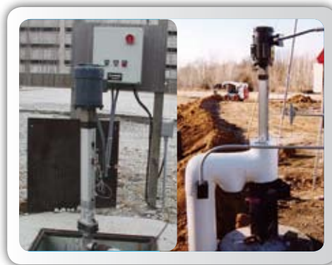
Pump in Coal-Tar Recovery Application
