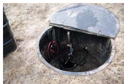
Blackhawk Pneumatic Anchor Pump pumping tar pitch.
