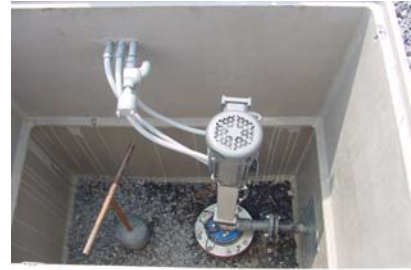
Explosion-proof Electric Anchor Pump and motor meet NEMA 4 classification.
