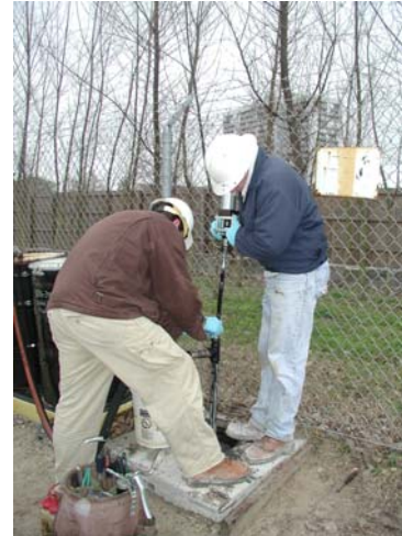
Because the coal tar is so thick, oily and sticky, the Blackhawk Trident pneumatic piston pumps are cleaned every night for top performance the next day.
