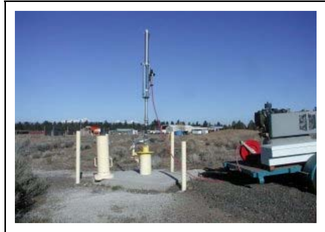
The controls on the top of the Blackhawk Anchor Pump 101A make it easy to install, inspect, trouble shoot, maintain and repair.
