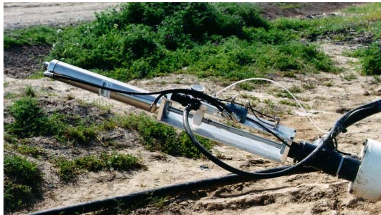
Close-up of the Side Slope Anchor Pump 102A manhole discharge
