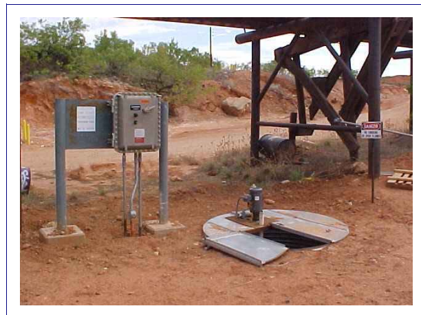
Blackhawk Explosion-Proof Electric Anchor Pump pumps old extremely flammable viscous petroleum byproduct 24 hours/day.
